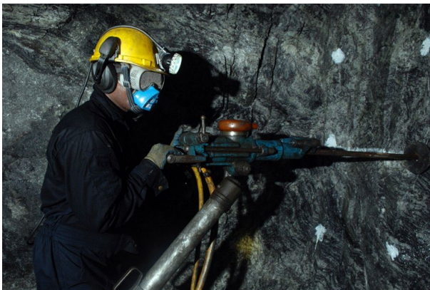
Drilling at underground
